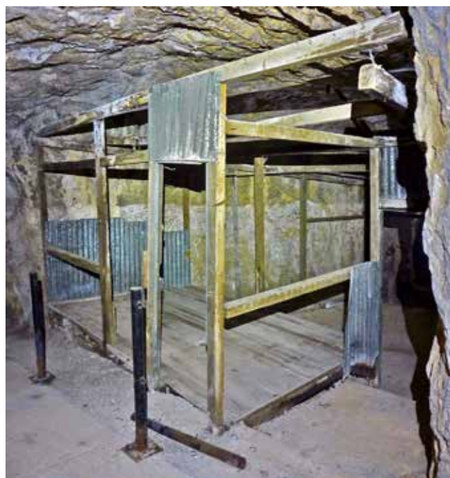
Queen's Gallery: SOE Wireless Station in an 18th-century Casemate
